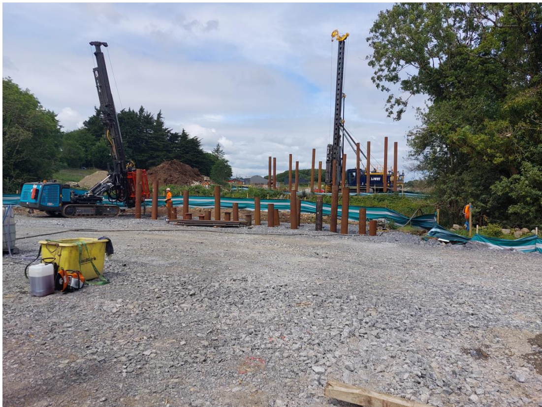
Driving of Steel Piles for ST07 Foundations – Lough Kip River Overbridge
