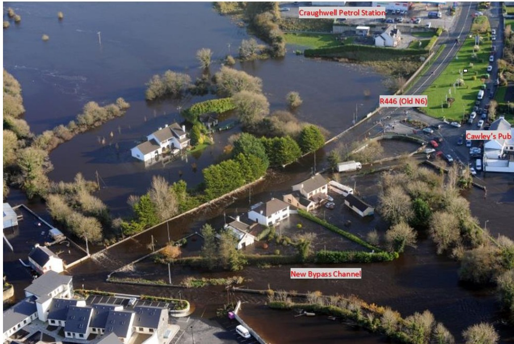
Flooding of November 2009
