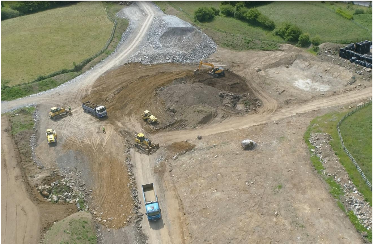
Earthworks operation ongoing at eastern Tie In
