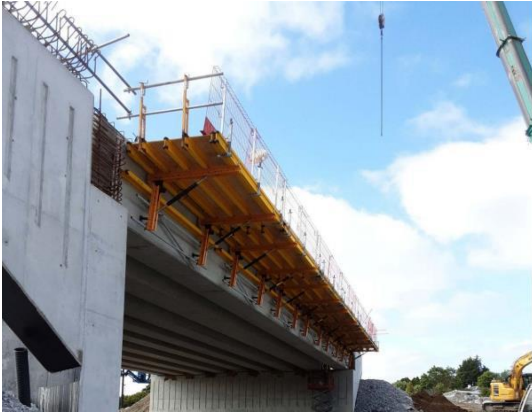
Works ongoing at Knockferry Road crossing
