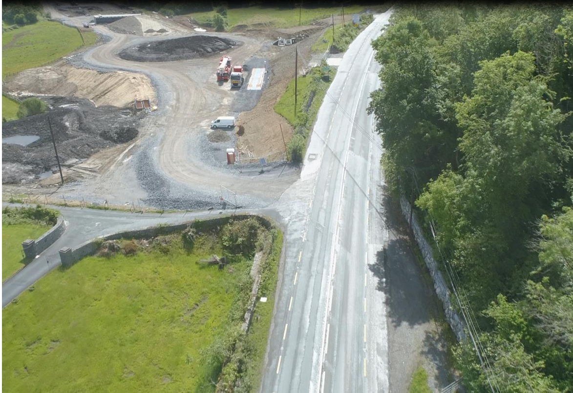
Location of Western Tie-In at Drimcong – Earthworks ongoing
