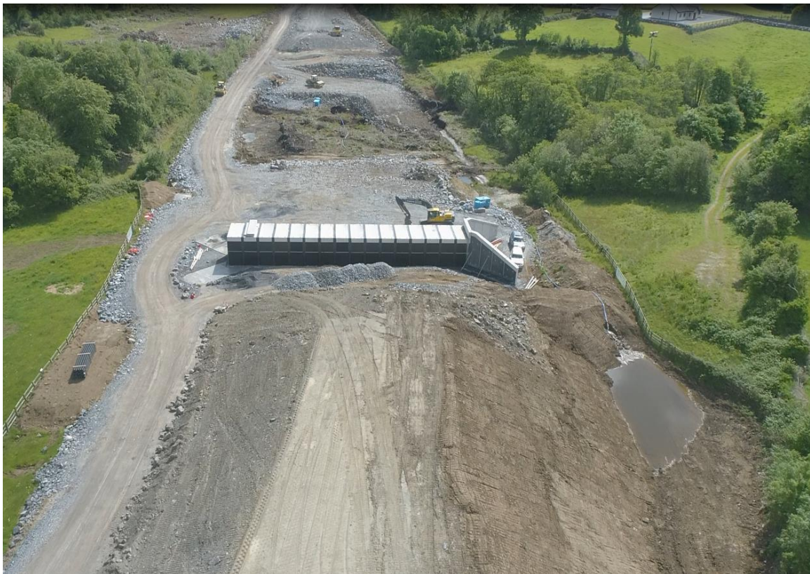
Construction works ongoing for ST02 a Farm Underpass at Killrainey
