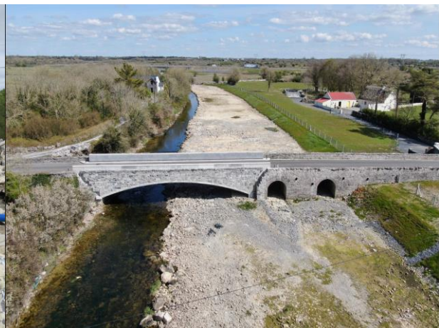
Completed works Dunkellin Bridge April 2021
